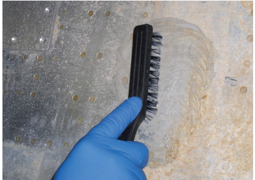
Figure 7-5-1. Removal of oil and surface dirt with bristle brush.
