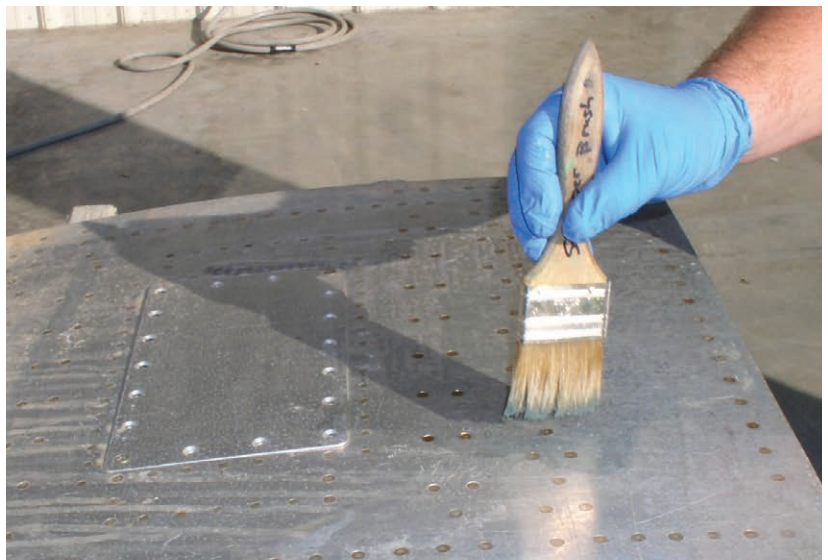
Figure 7-5-4. Treat corroded aluminum surfaces.
