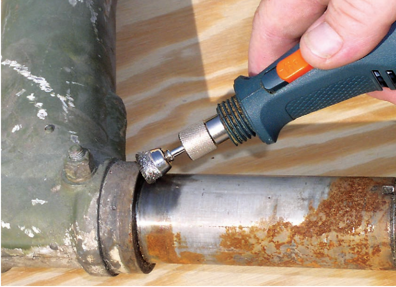
Figure 7-5-6. Mechanical removal of corrosion from steel surfaces.
