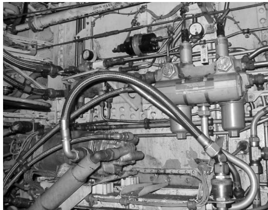
Figure 9-4-3. Hydraulic tubing and hoses in the main landing gear well of a Boeing 737 are particularly vulnerable to damage from stones, hail, and other debris.
