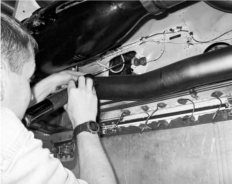
Figure 9-2-1. An AMT uses a flashlight and mirror to inspect inside a panel in the cramped conditions of an air conditioning bay.
