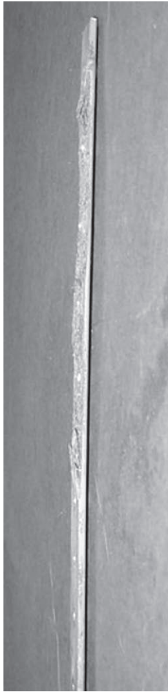
Figure 9-8-6. An example of exfoliation corrosion on a stringer section. The corrosion products have more than doubled the part's original thickness.
