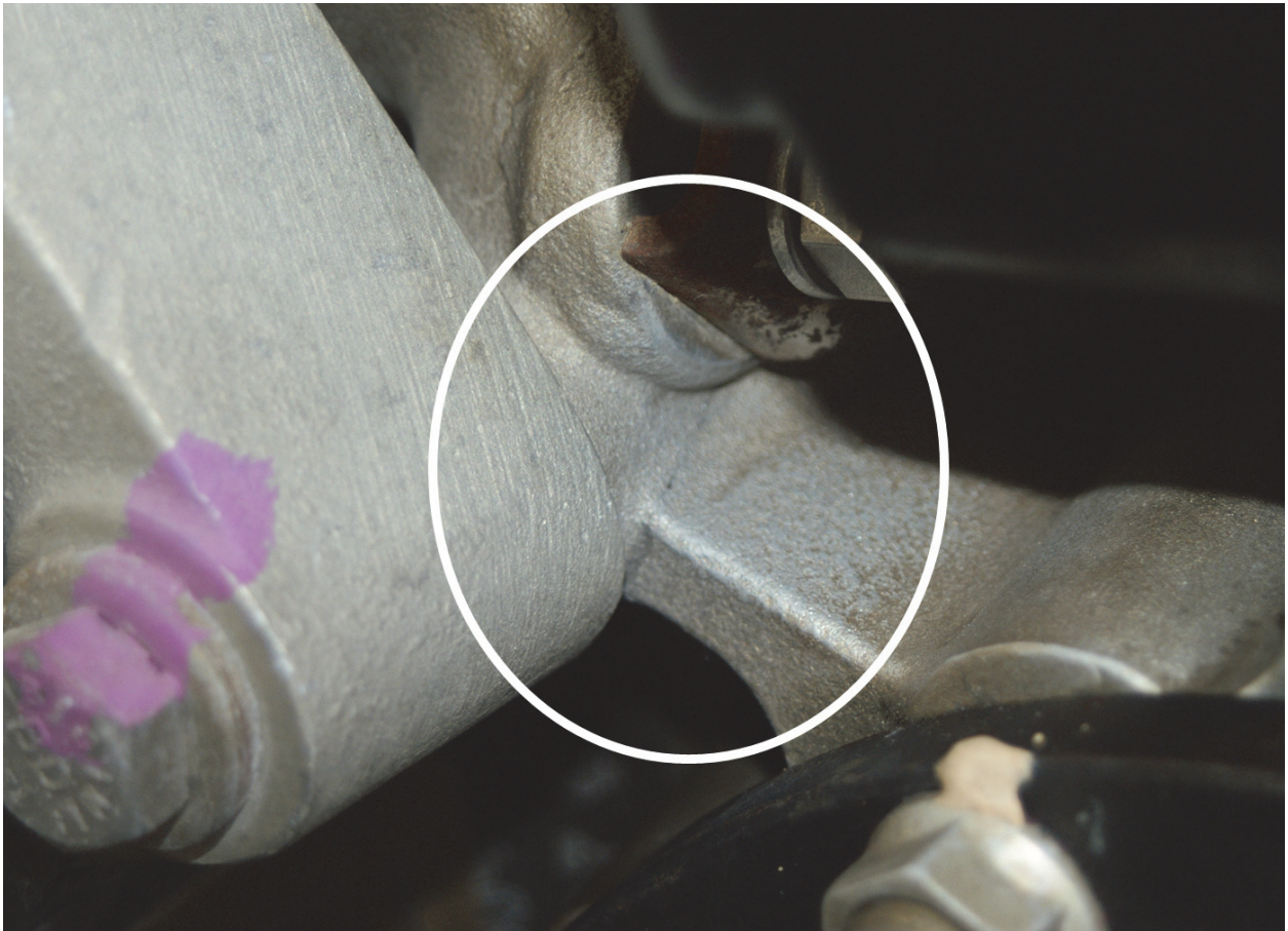
Figure 6-47. Suspect Crack Indication
