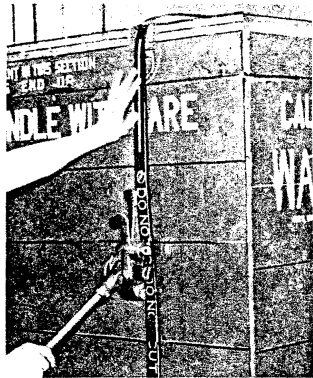
Figure 4-41. Tightening Steel Straps
