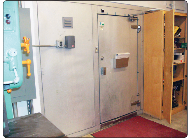
Figure 7-44. Walk-in freezer for storing prepreg materials.
