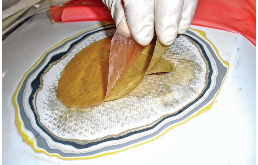
Figure 12-7-10. The patches are cut to size noting the weave direction, and a layer of peel ply is placed over the repair.
